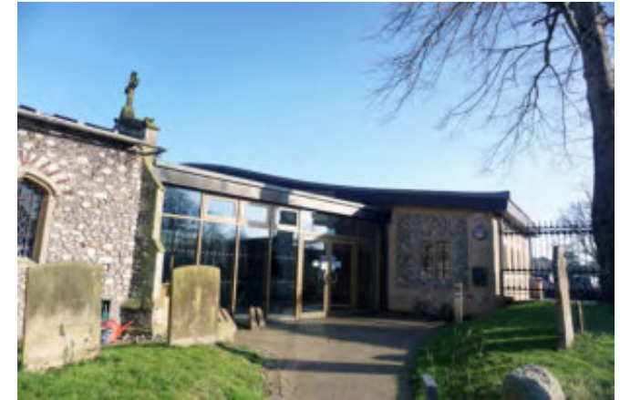
Extension to St. Andrew's Church
