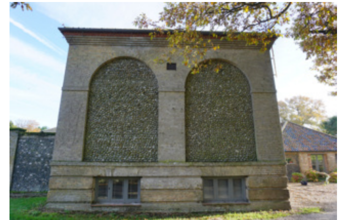
The north elevation of the tun house, with stock brick decorative details and arched flint recesses
