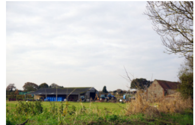
Modern barn seen from The Street
