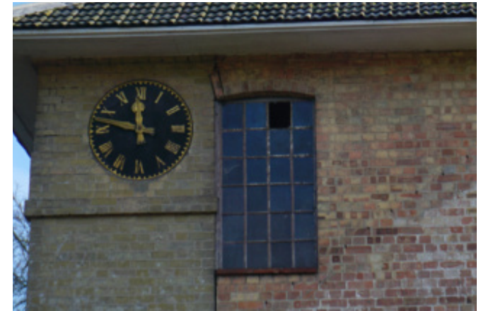
Rusting window frame with glass pane missing
