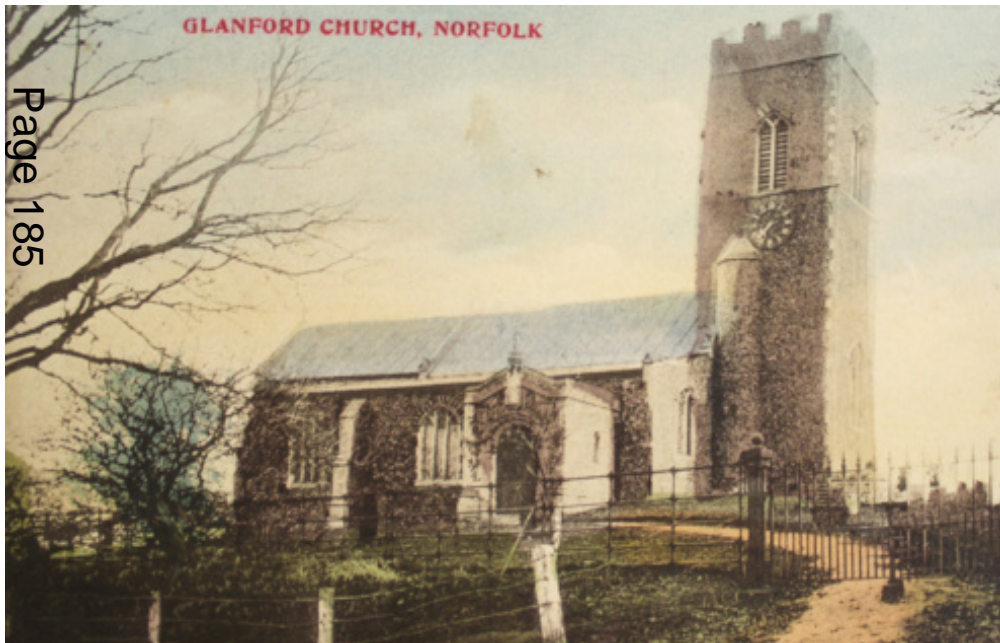
View of Glandford Church showing the iron boundary fencing, which remains in part today (Norfolk Record Office: C/GLA) **Permission pending**
