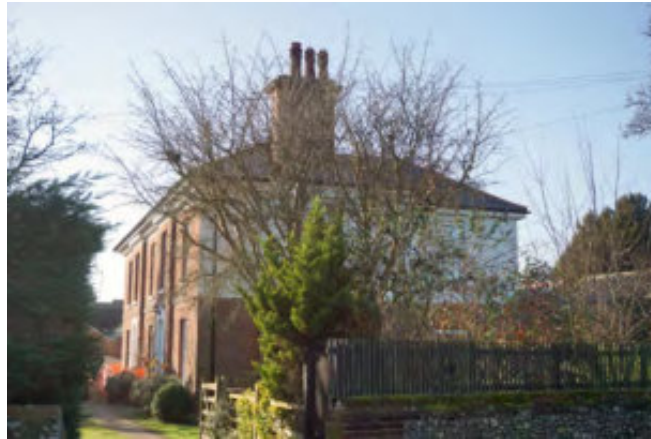
Converted Police Station on Station Road
