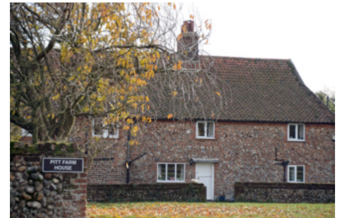
The farmhouse at Pitt Farm
