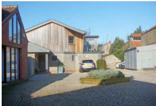
Morston House on Jacob's Place
