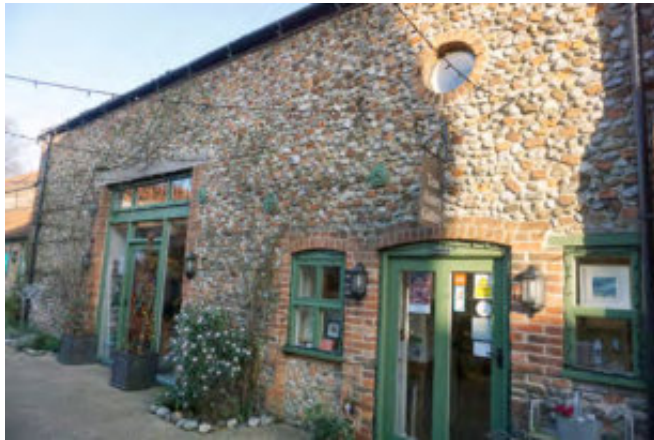
Converted outbuildings on Hooper's Yard
