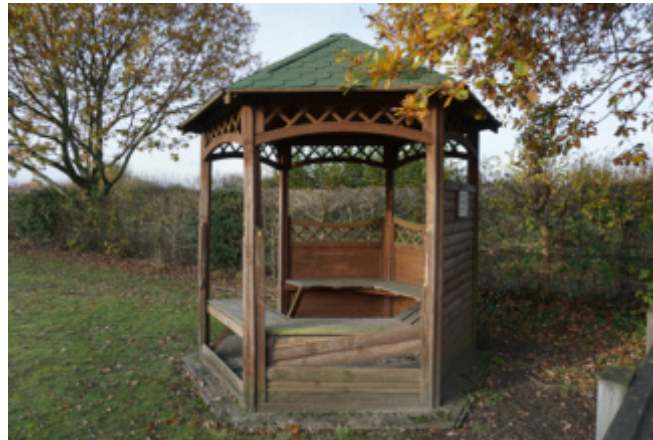
Damaged shelter at the playground
