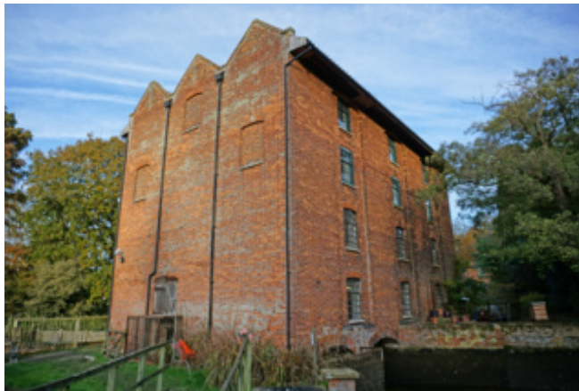
Letheringsett Mill, west and south elevations
