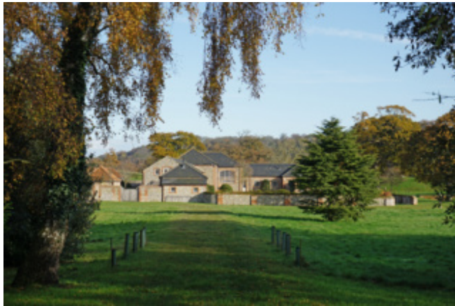
Large scale buildings at Hall Farm
