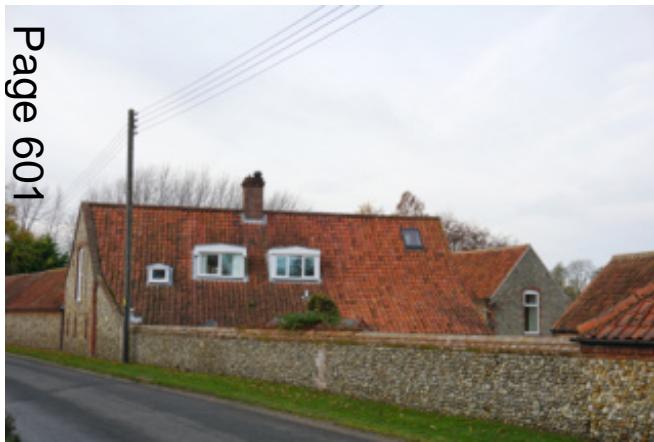
Converted barn at Home Farm
