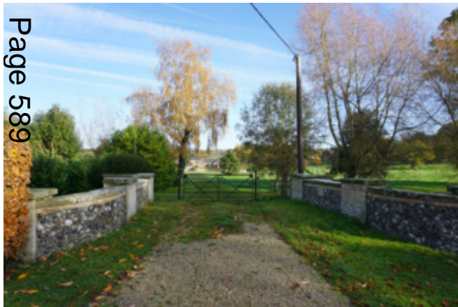
Flint, brick stone walls to a bridge leading to the south-west entrance to Hall Farm from Church Lane, with metal park fencing and gates
