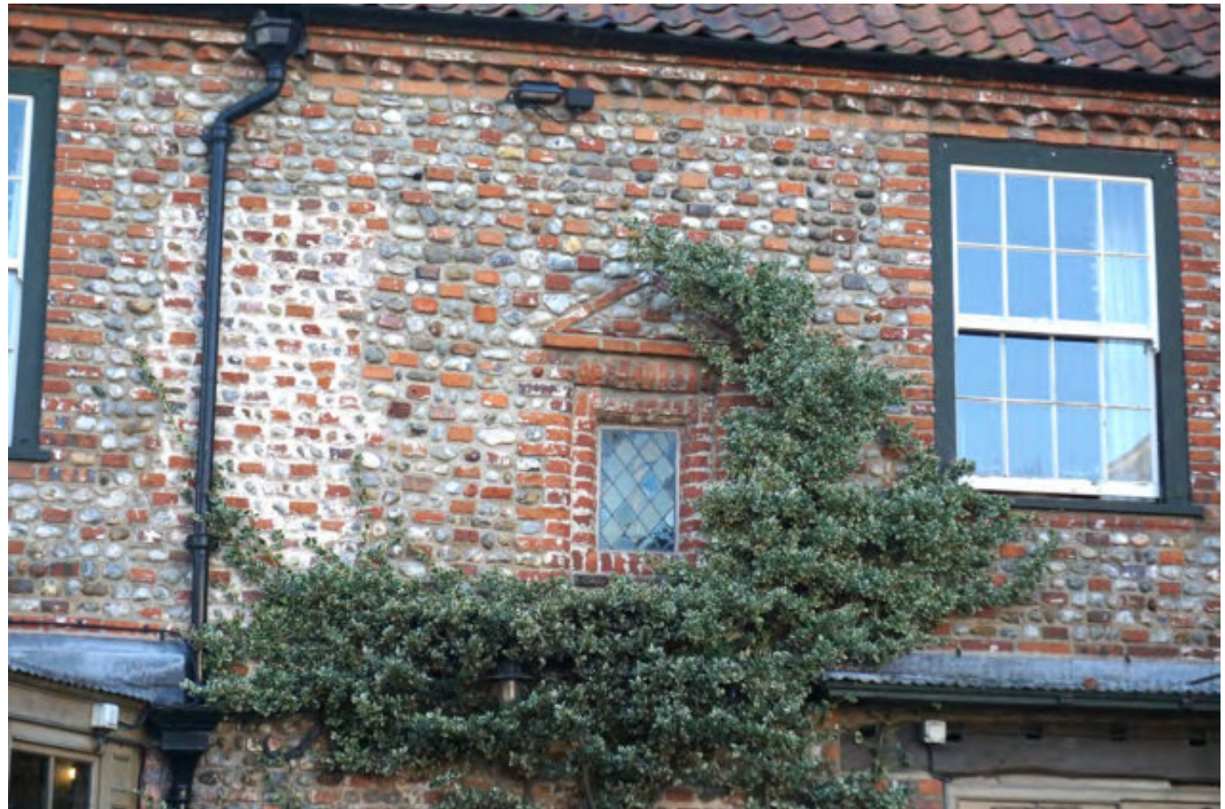
Flint and brick chequer pattern and small sixteenth century window on Byfords, Shirehall Plain
