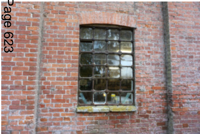
Rusting and bowed window on the mill
