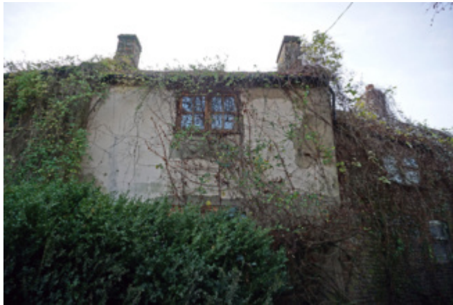
Cementitious render repairs
