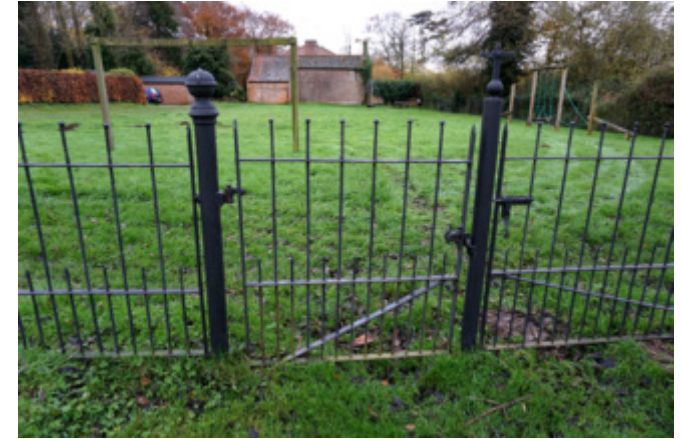
Metal gate and railings to the graveyard
