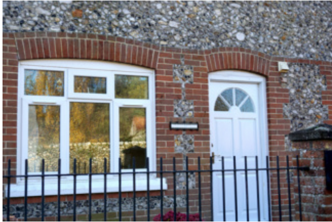
uPVC window and modern replacement door
