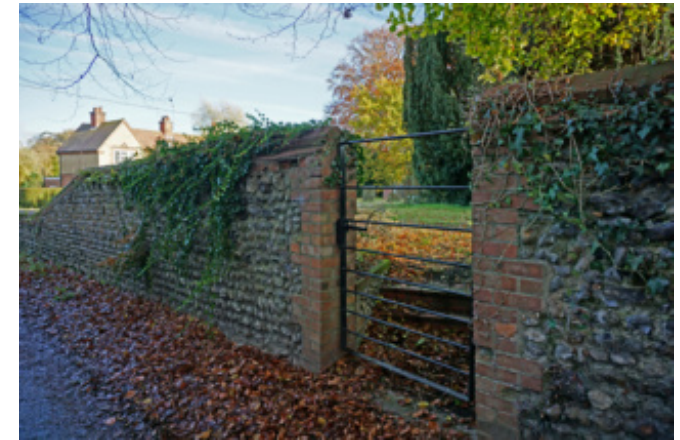
Flint wall and metal gate to the churchyard
