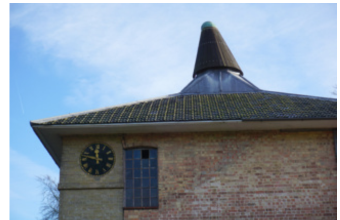
The distinctive roof of the former malt kiln, with the Coronation Clock on the west elevation
