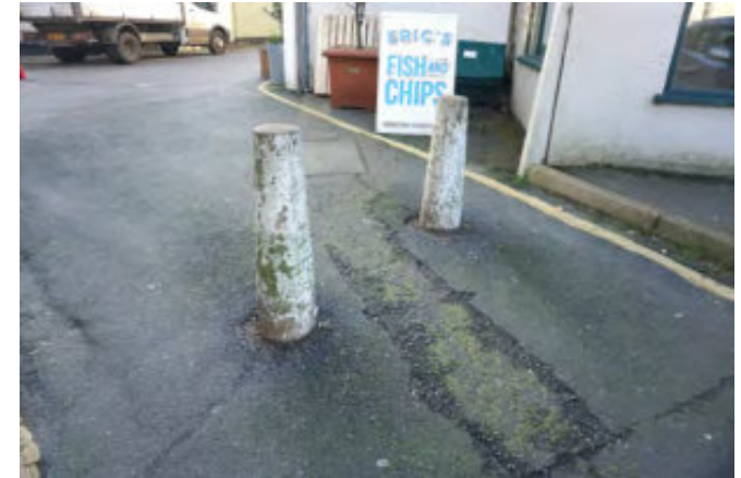
Unattractive concrete bollards with peeling paint
