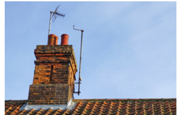
Eroding brickwork on a chimney
