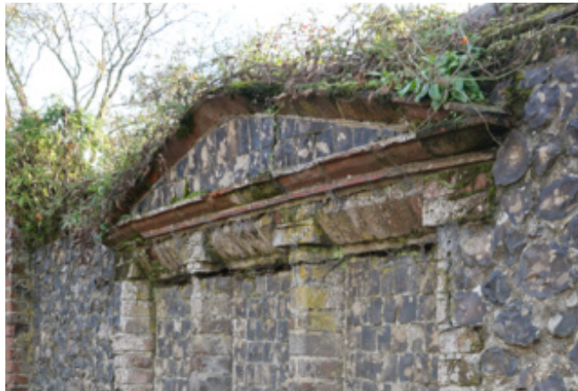
Vegetation growth on the pedimented feature on Holt Road
