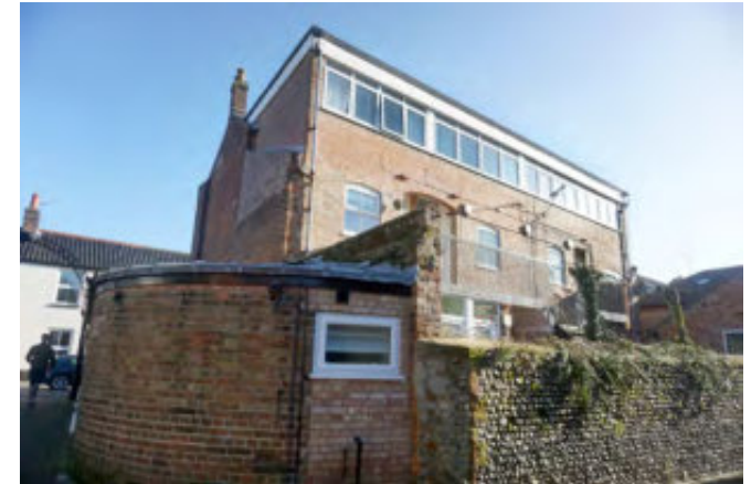
Poor quality extension as seen from Lion House Court
