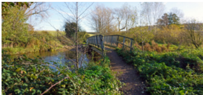
The bridge over the ford
