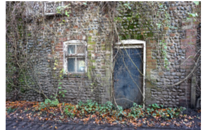
Timber work in poor condition
