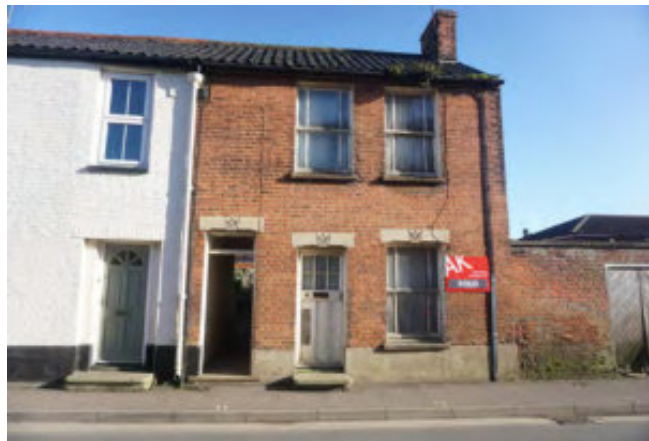
Vacant property on New Street
