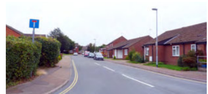
Modern housing to the south of the Conservation Area boundary
