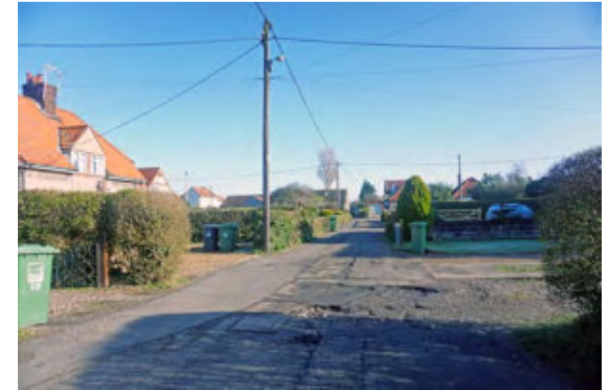
Poor surfacing of The Fairhaven
