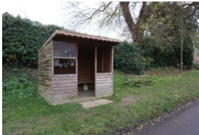
Bus shelter in poor decorative condition
