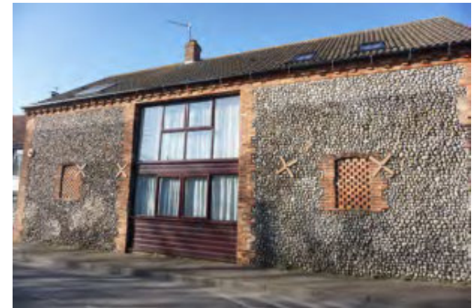
Converted barn on Valley Lane
