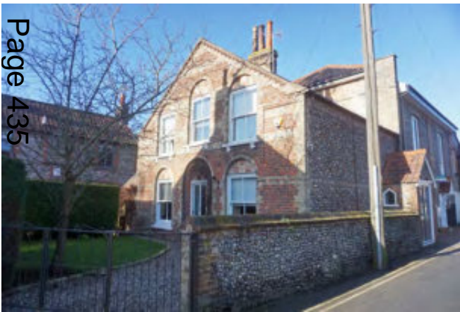
Converted Corn Hall on Albert Street
