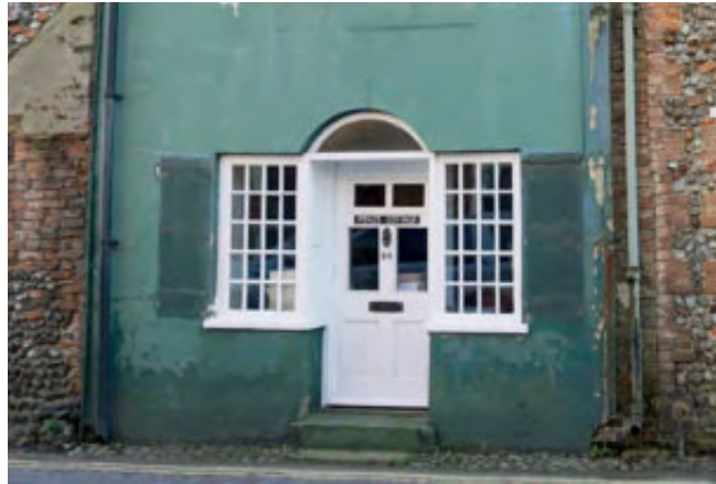
Poor condition of paintwork
