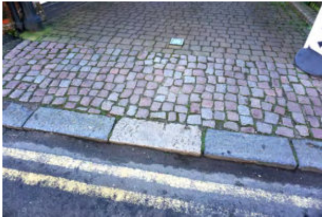
Granite kerb stones, granite setts and brick pavers on New Road, with double yellow lines
