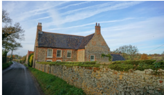
Meadow Farmhouse, with Georgian sash windows inserted into an earlier building
